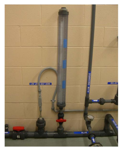
Figure 2-6. Alum Pump Calibration Chamber.
