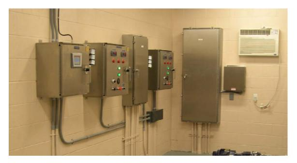
Figure 2-4. Overview of Alum System Control Panels.
